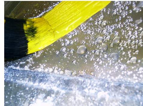
Applying RA 500M on a completely wet substrate
