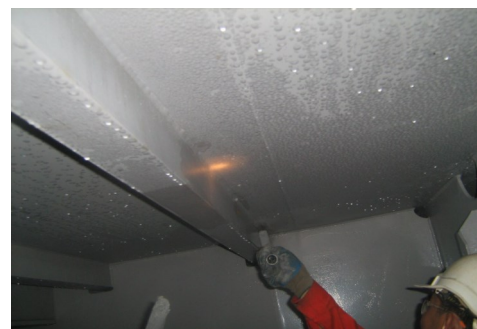
Applying RA 500M on a wet surface in a ballast tank
