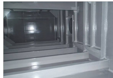
RA 500M applied in a potable water tank
