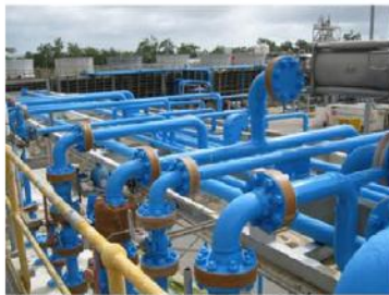
After – Coated Pipework
