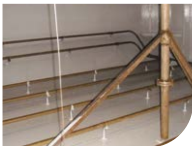
Crude Oil Tank
