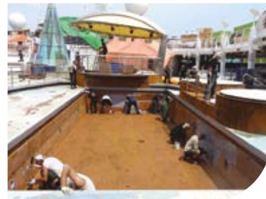
Applying Primer to Mechanically Prepared Swimming Pool
