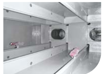
Sea Water Ballast Tank
