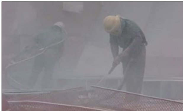
Abrasive blasting creates high levels of dust. Photo courtesy of NIOSH.
