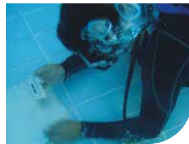
Filling swimming pool tile cracks
