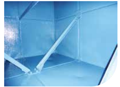
Potable Water Tank
