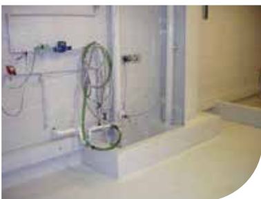
Damp-crete™ RH 800 Concrete Bund Repair
